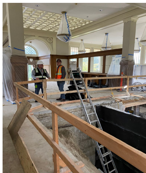
Green Lake Seismic Retrofit Project
