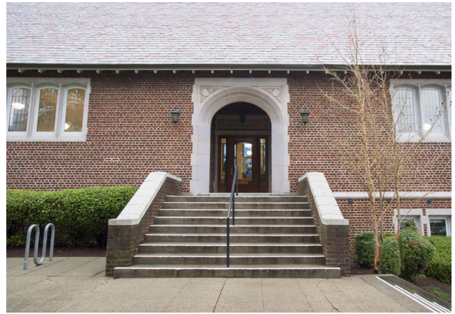
New roof at Queen Anne Branch
