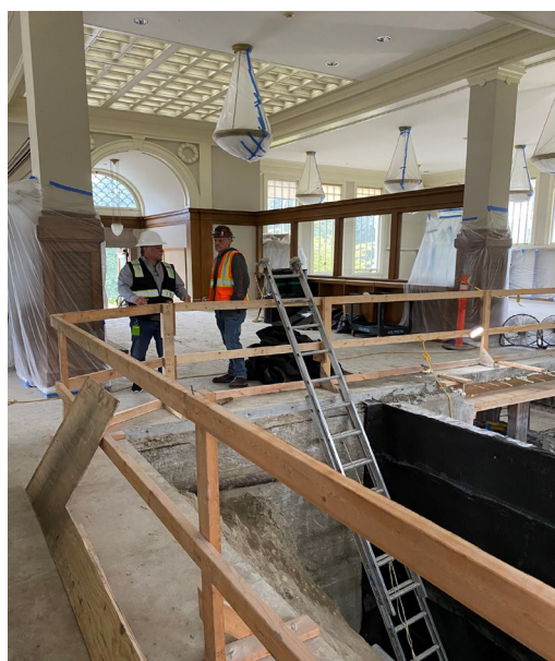
Green Lake Seismic Retrofit Project
